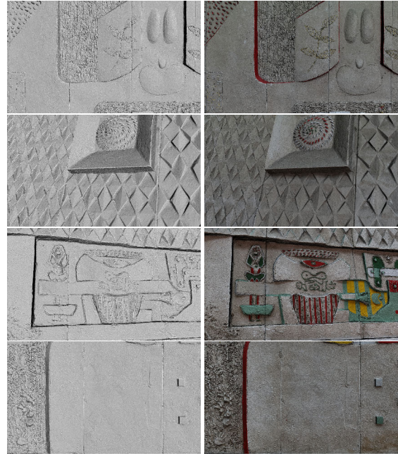
Figure 3: 3D model details. The 3D model captures the different surface textures, derived from the various sculpting techniques used by Nivola. Some traces of the sculpting process are visible using the virtual grazing light.
